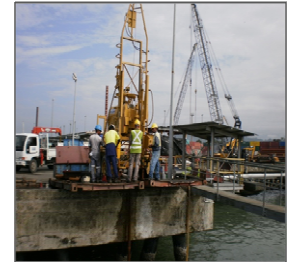
Geotechnical Drilling: Lae Wharf
