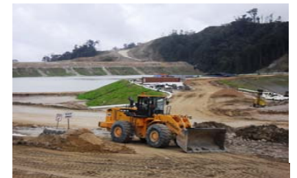
Civil Works on Dam at Hidden Valley Gold Mine:- MMJV
